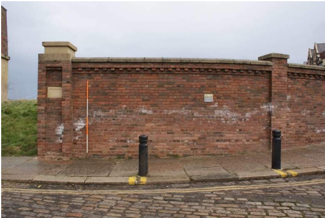
Plate 8 Rebuilt southern wall (Section A1), looking north
