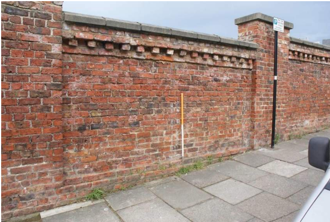
Plate 12 Wall section (B4), looking north-west
