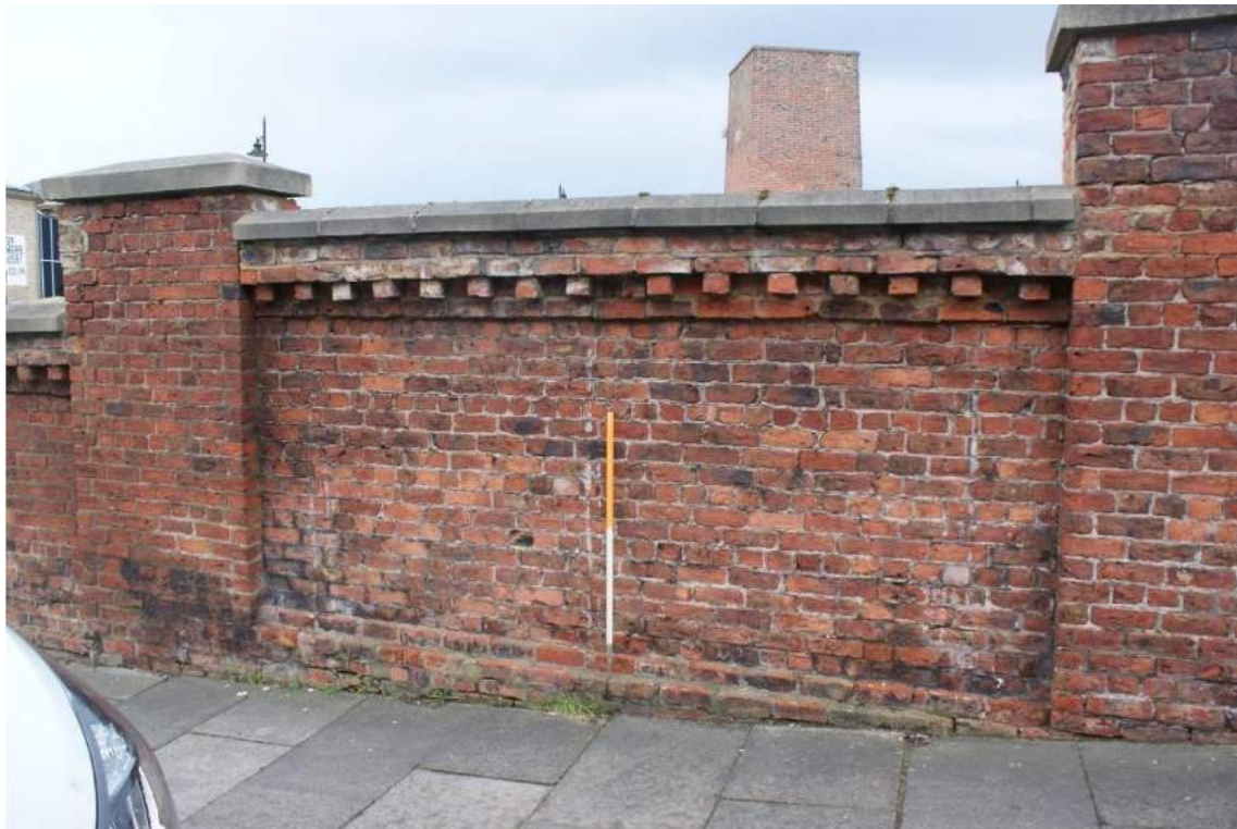
Plate 10 Wall section (B2), looking north-west
