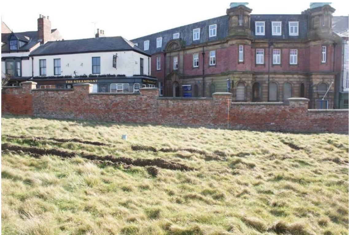
Plate 19 Rear elevation of Section B (B3 to B6) looking south-east
