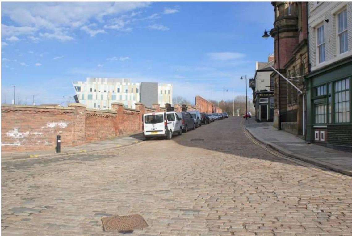
Plate 2 Mill Dam Wall, looking north along Mill Dam
