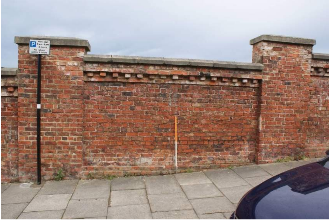
Plate 13 Wall section (B5), looking north-west
