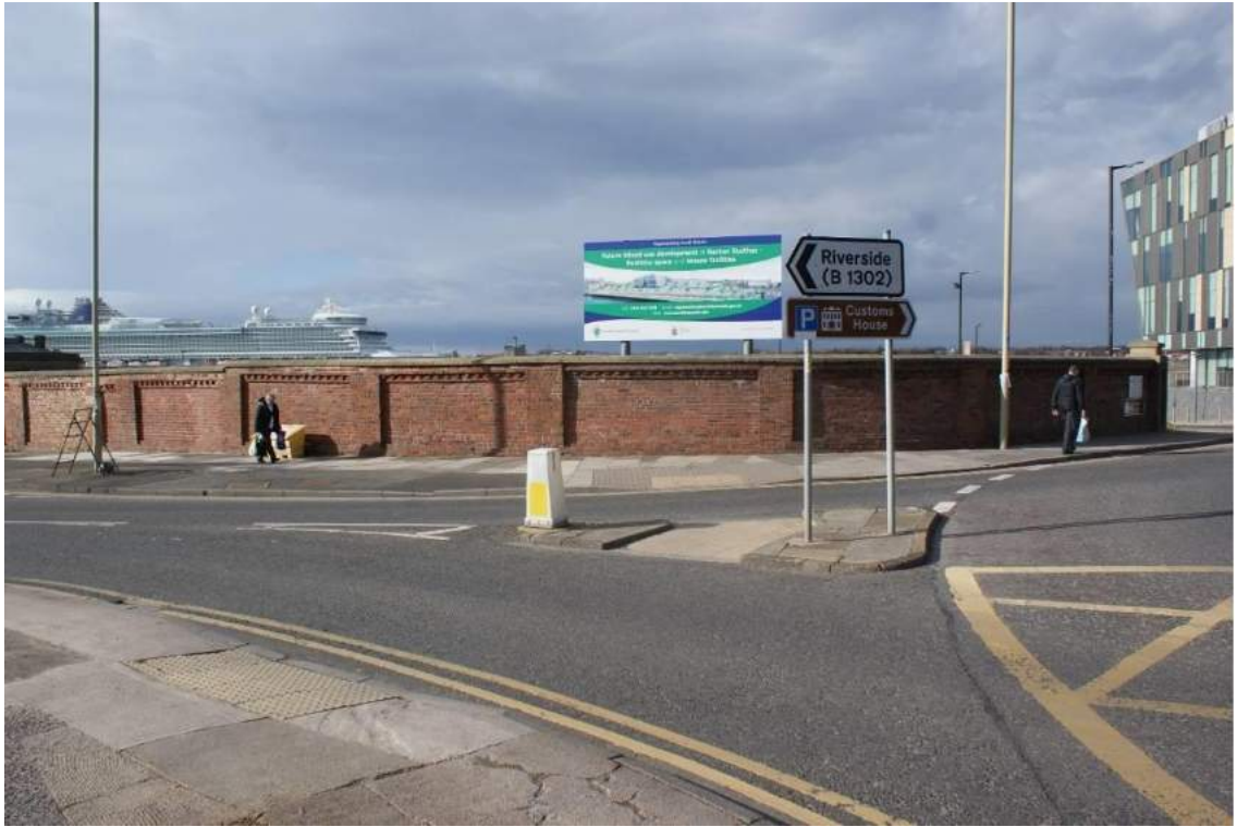
Plate 4 Northern end of Mill Dam Wall, looking west toward Harton Quay
