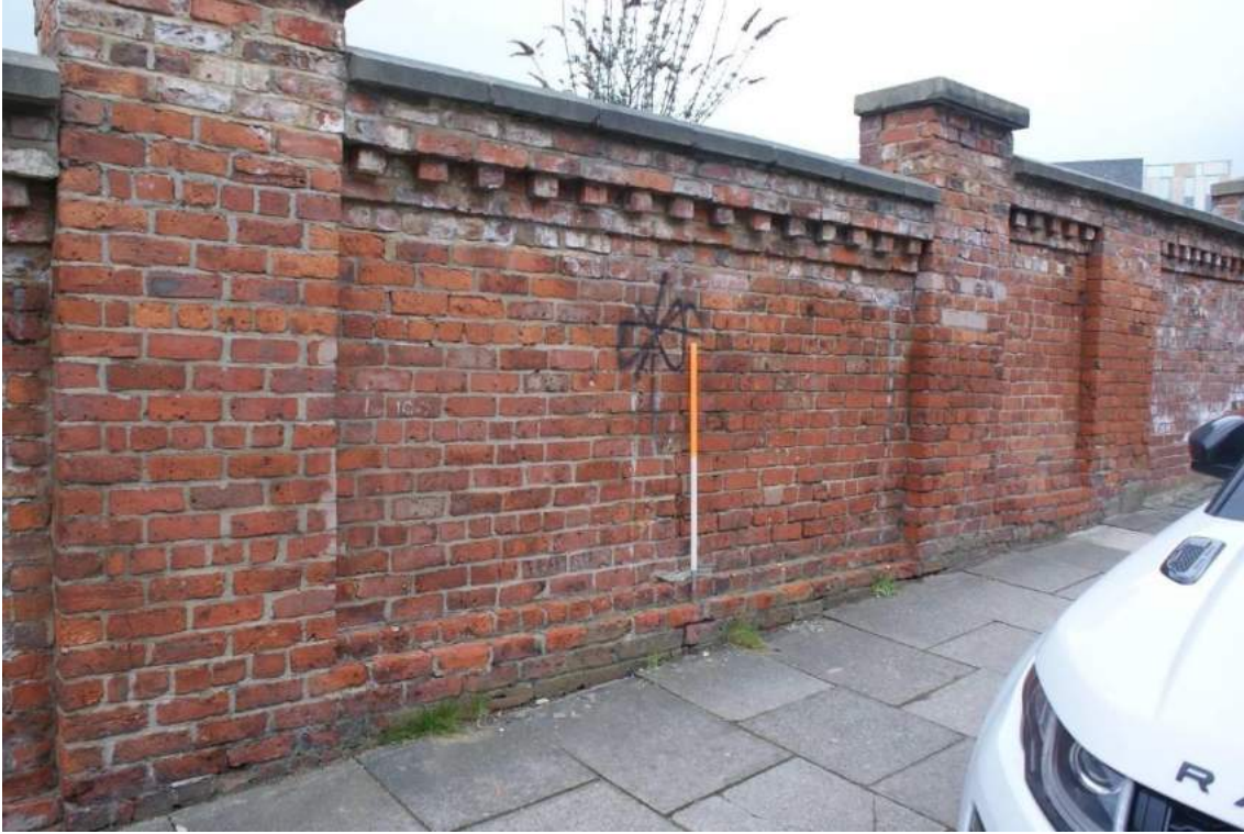
Plate 15 Wall section (B7), looking north-west
