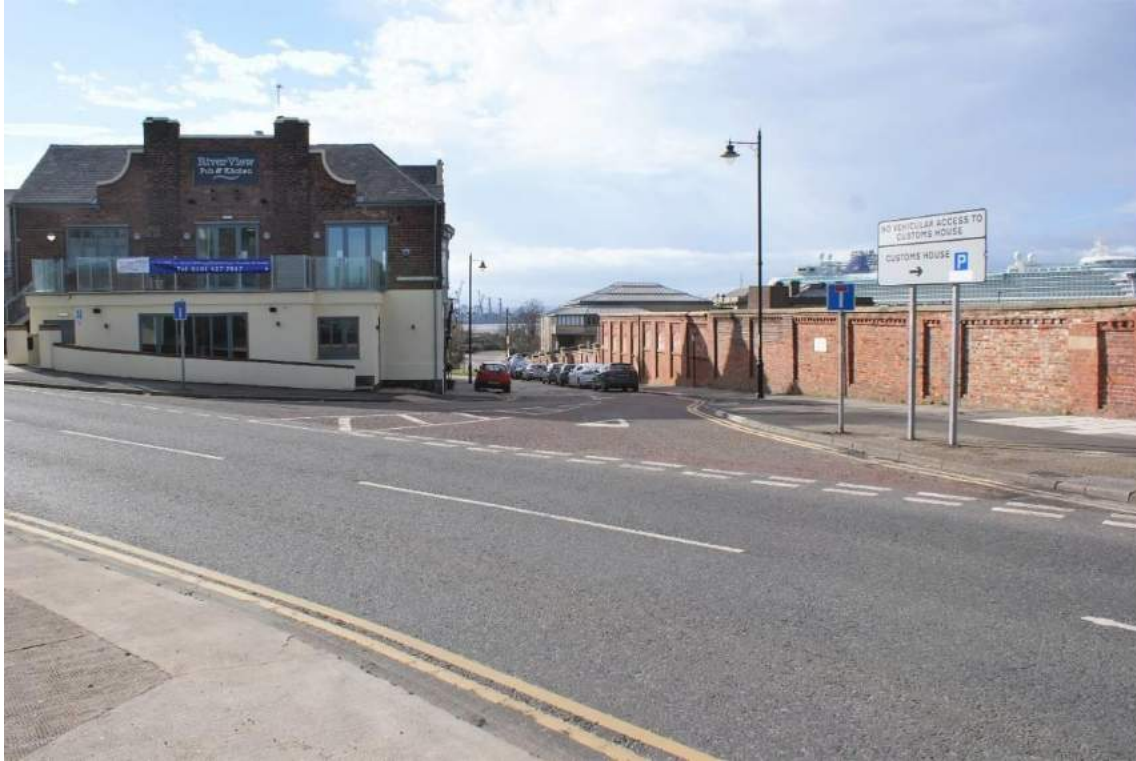
Plate 3 Mill Dam Wall, looking south along Mill Dam
