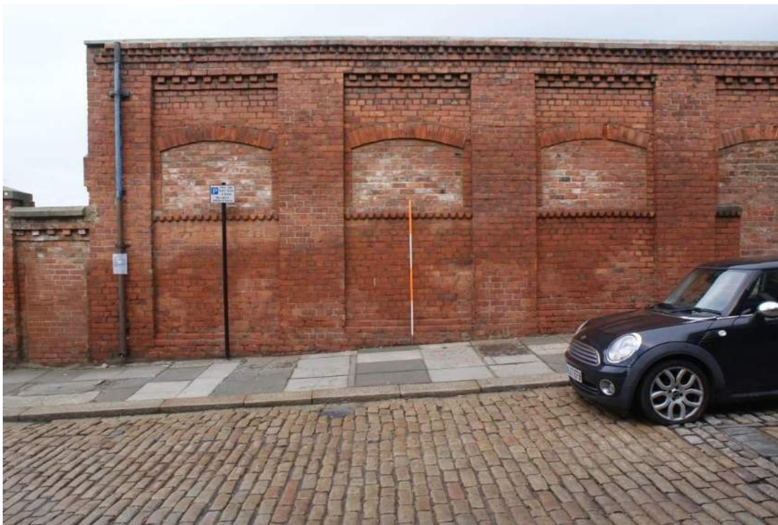
Plate 21 Section C, southern bays to façade, looking north-west
