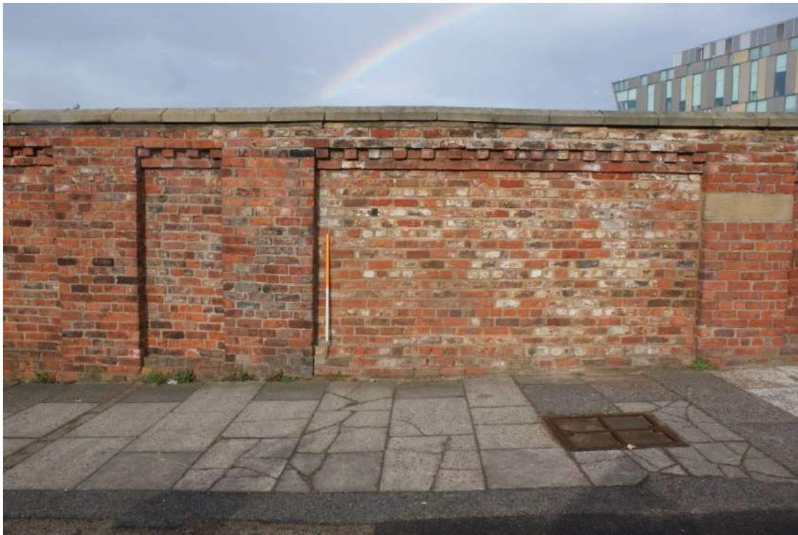
Plate 29 Blocked former entrance opening (D5), looking
