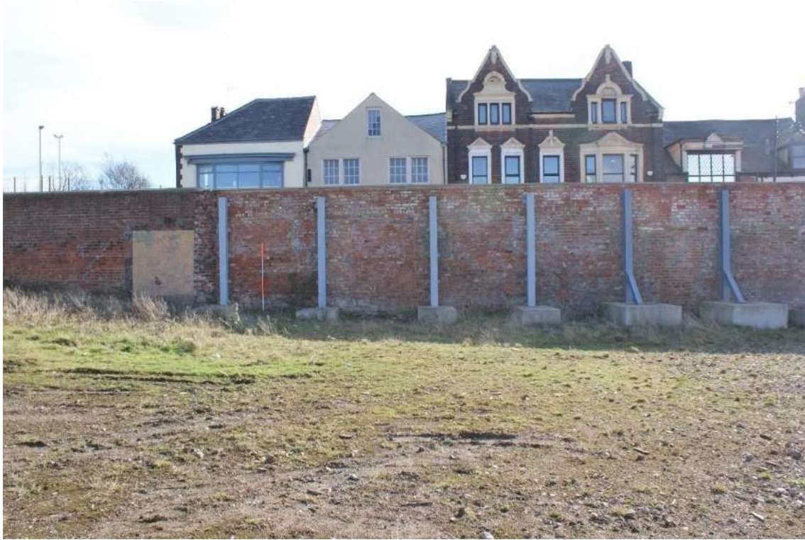
Plate 26 Rear elevation of Staithe House façade (C), north end, looking south-east
