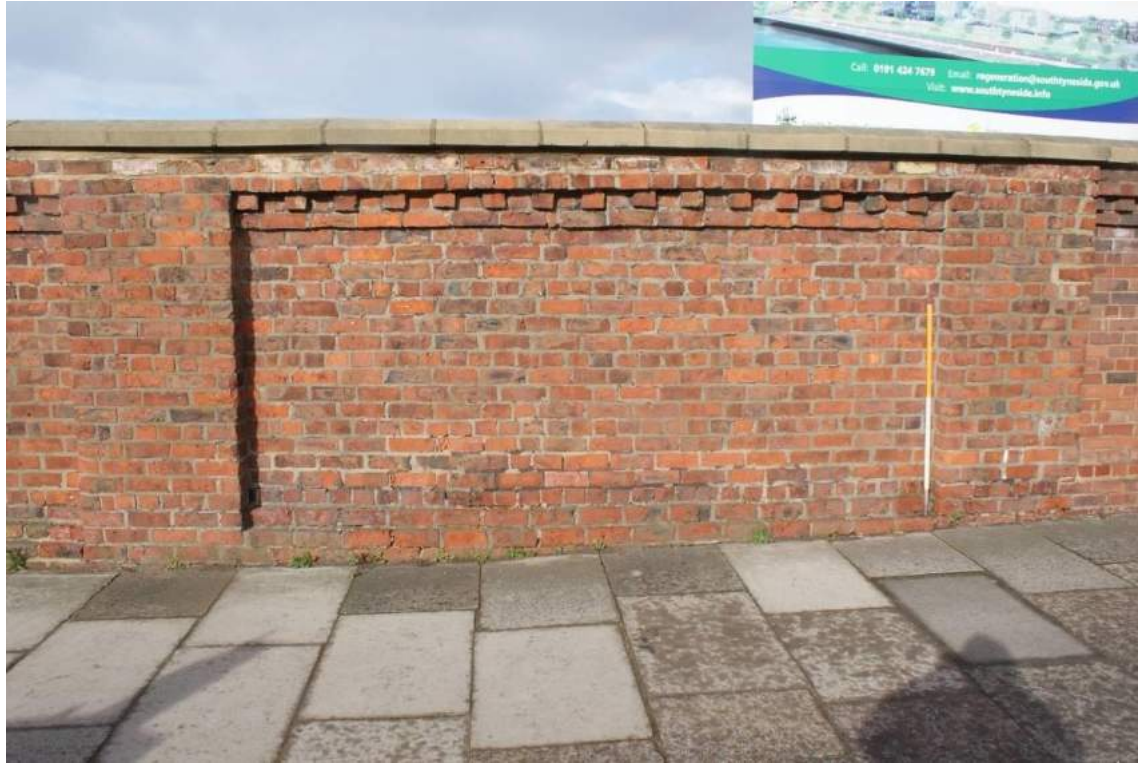
Plate 32 Wall Section (D8) looking north-west
