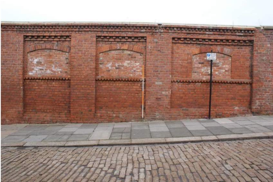
Plate 24 Section C, northern bays, looking north-west
