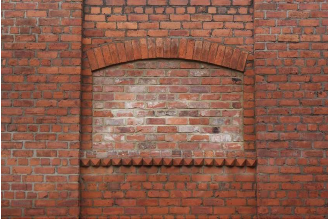
Plate 22 Section C, detail of blocked window opening
