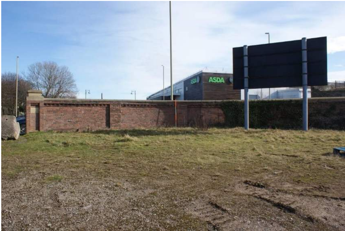
Plate 35 Rebuilt northern section (E), looking north-east
