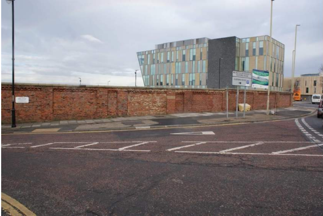
Plate 30 Wall Section (D) looking north-west
