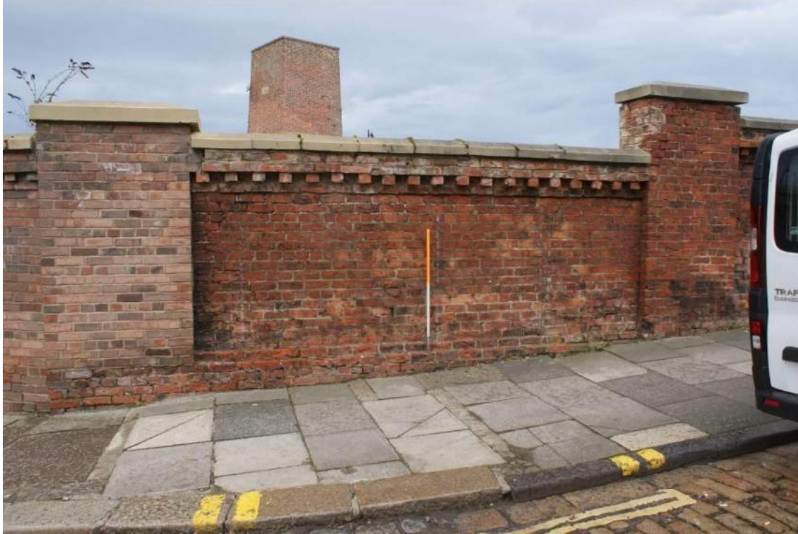
Plate 9 Wall section (B1), looking north-west
