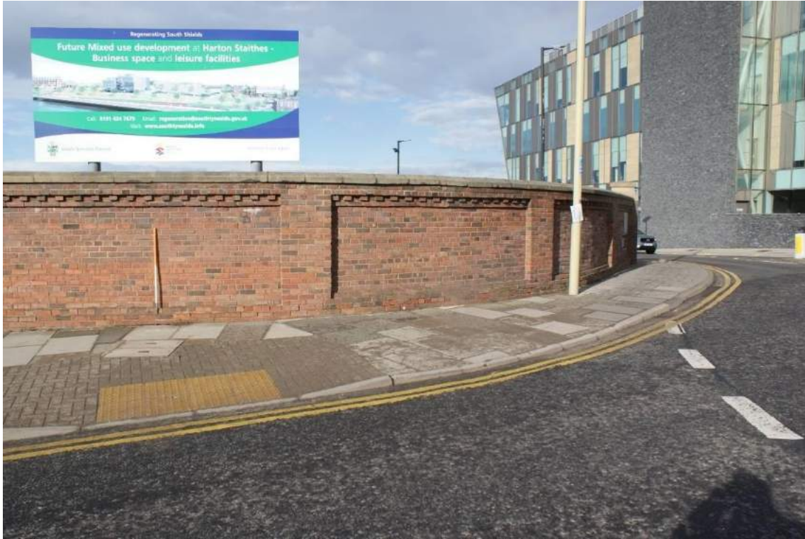
Plate 34 Rebuilt northern section (E), looking north-west
