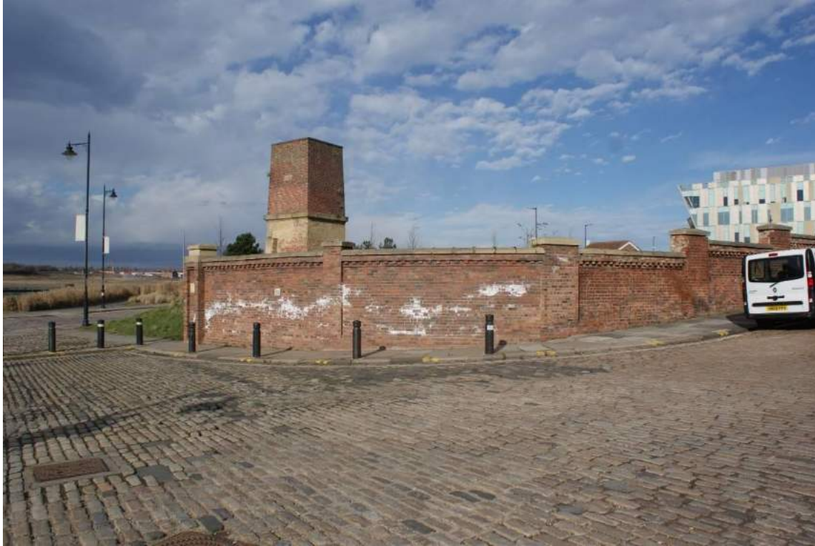
Plate 1 Mill Dam Wall, Rebuilt southern end of wall, looking north-west
