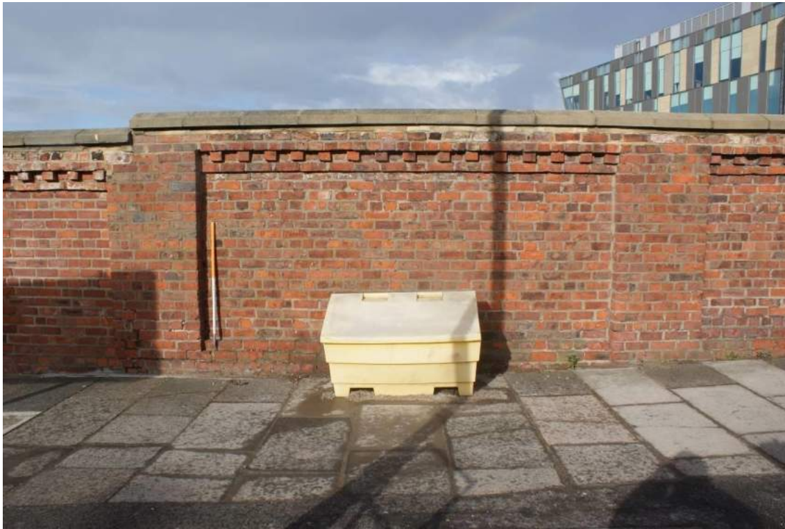
Plate 31 Wall Section (D7) looking north-west
