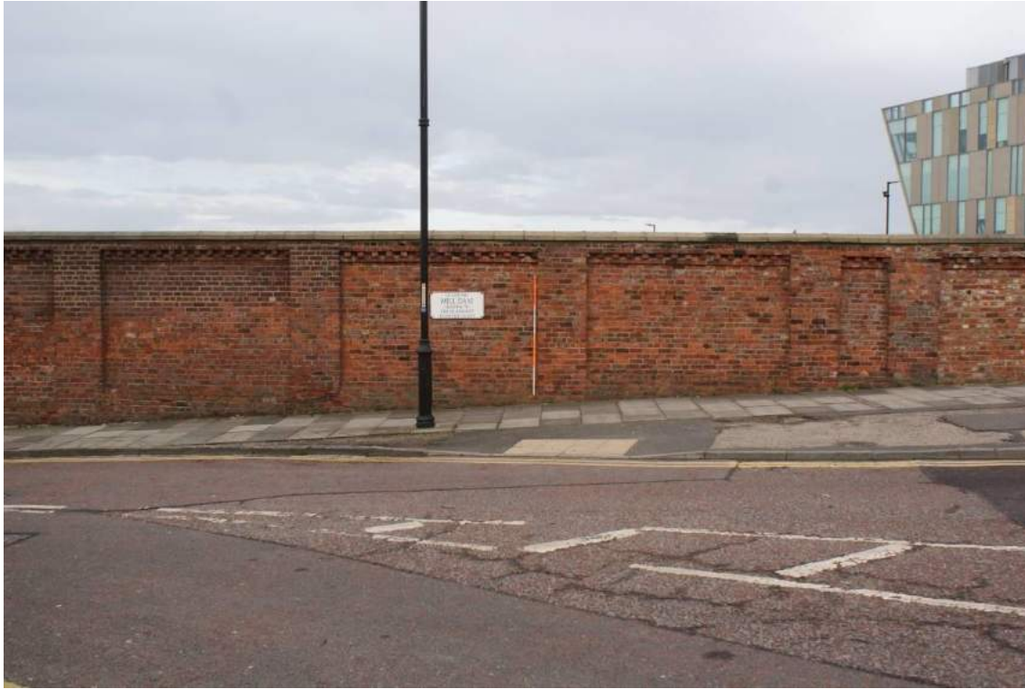
Plate 28 Wall Sections (D3 and D4) looking north-west
