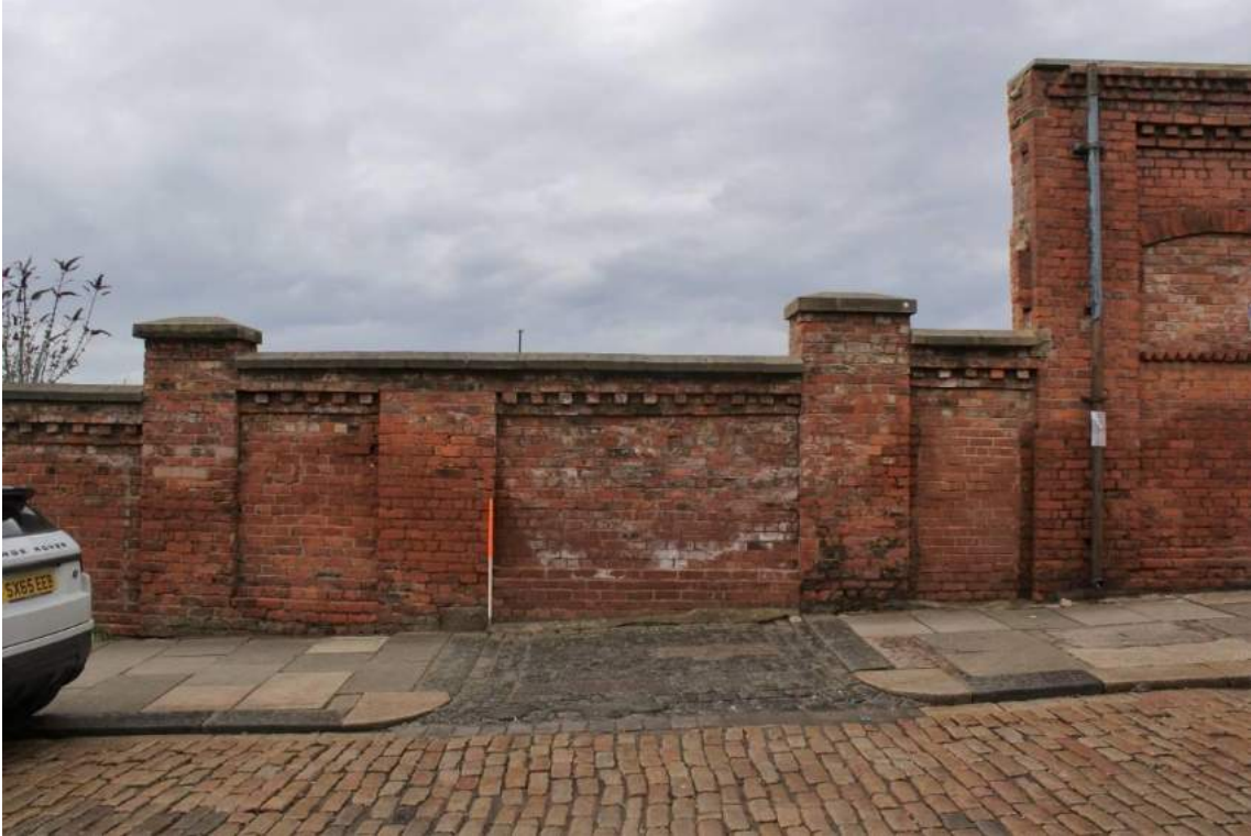
Plate 16 Former entranceway (B8) looking north-west
