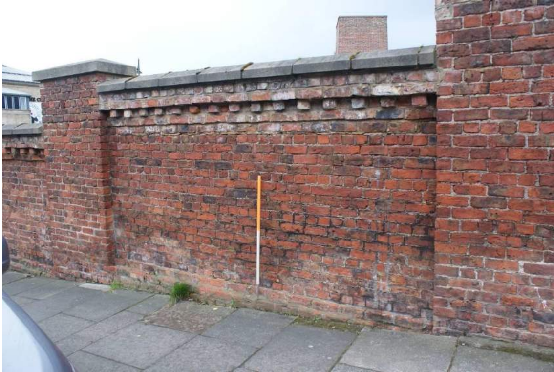
Plate 11 Wall section (B3), looking west
