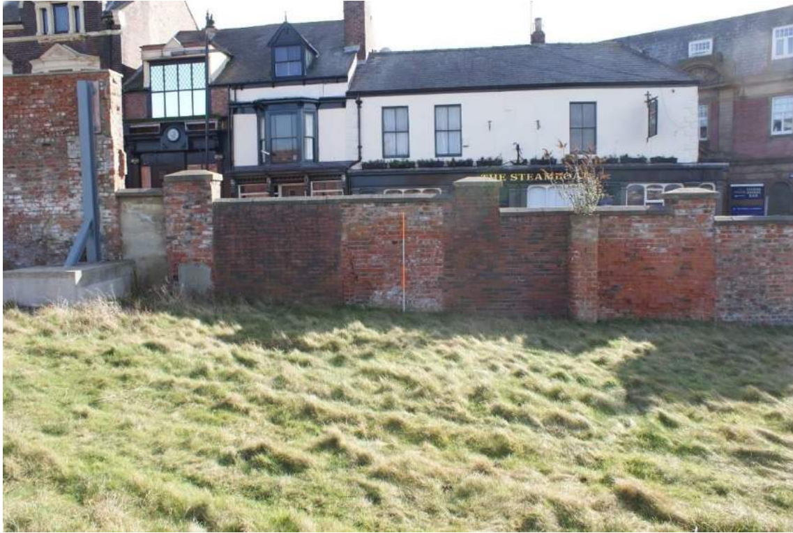
Plate 18 Blocked entranceway (B8) looking south-east
