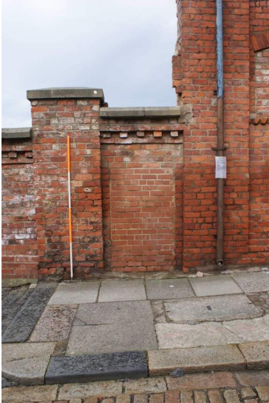
Plate 17 Blocked door opening (B9), looking north-west
