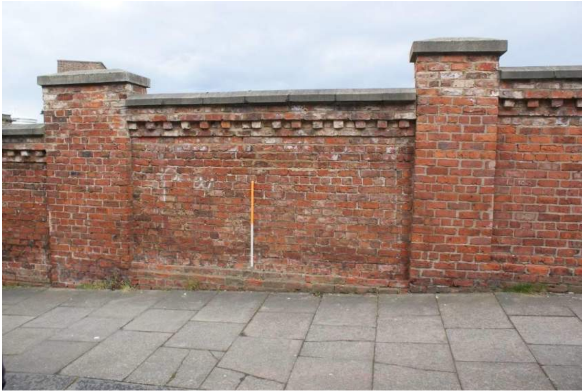
Plate 14 Wall section (B6), looking north-west
